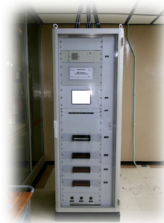
Fig. 1. DFRPM unit in operation in Itaipu Hydroelectric power plant.
